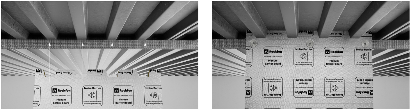
Top of Rockfon Plenum Barrier Board castle-cut to fill the flutes of the metal deck.
