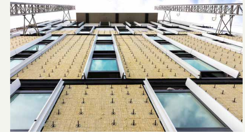
A stone wool insulation effectively works against temperature and noise
