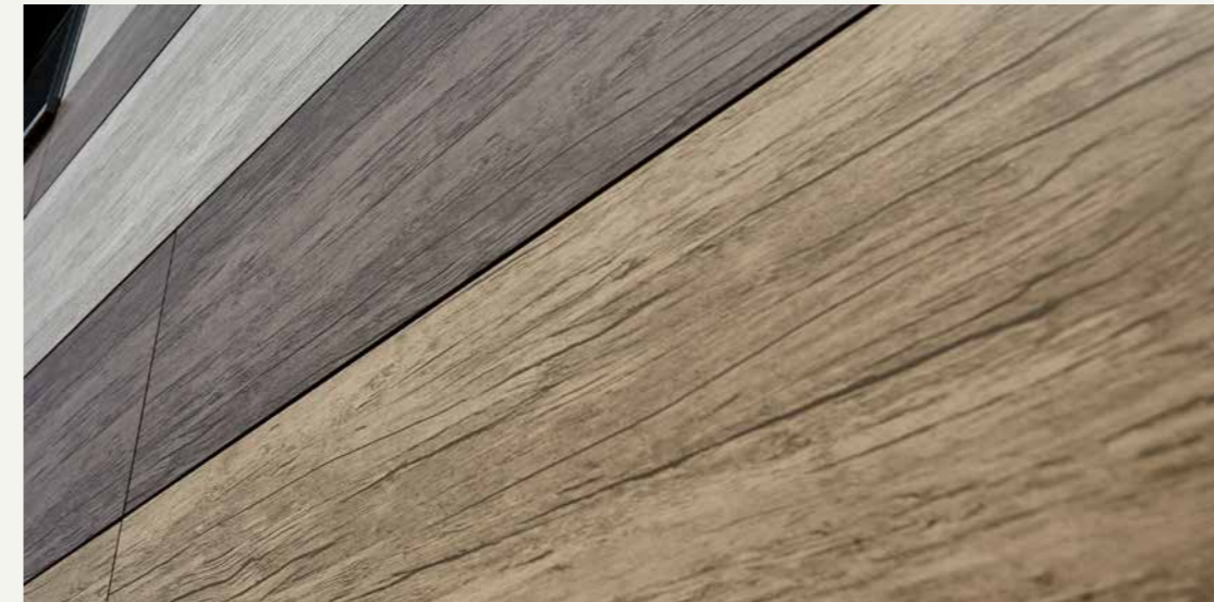
Concealed fixing - not visible from the outside
