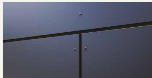
2. HPL and fibre cement boards: Joints need to be at least 10 mm wide.
