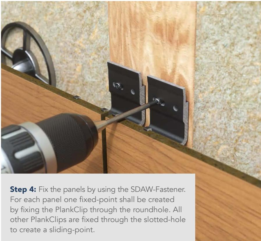
**Step 4:** Fix the panels by using the SDAW-Fastener. For each panel one fixed-point shall be created by fixing the PlankClip through the roundhole. All other PlankClips are fixed through the slotted-hole to create a sliding-point.
