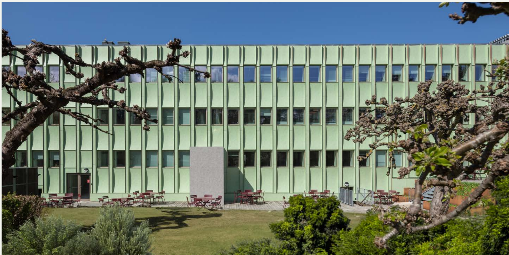
ROCKWOOL Nordics, Hedehusene, Denmark
